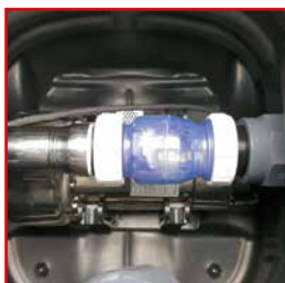
Check valve RSK and drain pump
